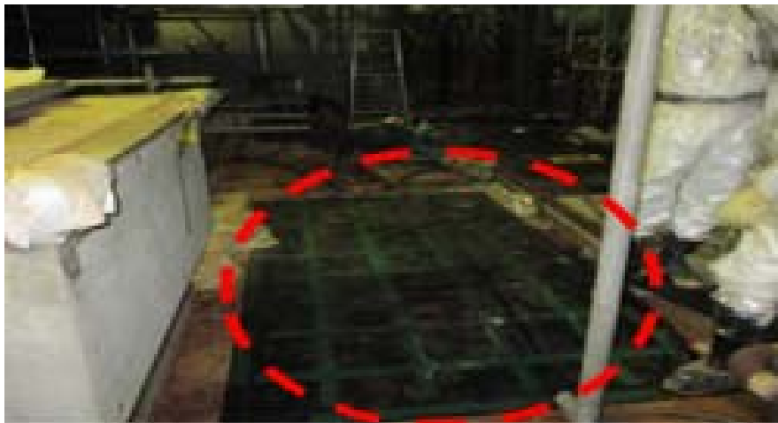
\beta -ray shielding by rubber mats
