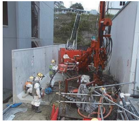
Exposure reduction measure: Placing L-shaped protection walls at the work area (Radiation source: left side building).
