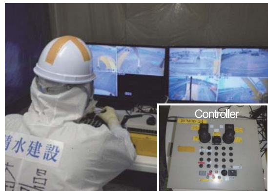
Exposure reduction measure: Topsoil stripping was conducted by a remotely operated RCM in high radiation areas.
