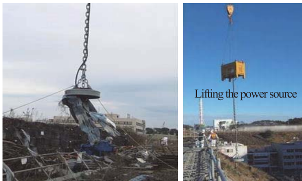
Exposure reduction measure: Using lifting magnets for efficient removal of high radiation debris on a slope.
