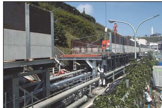
Exposure reduction measure: Installation of working platforms and RC shielding plates (air dose rate has been reduced to 1/4 – 1/3).
