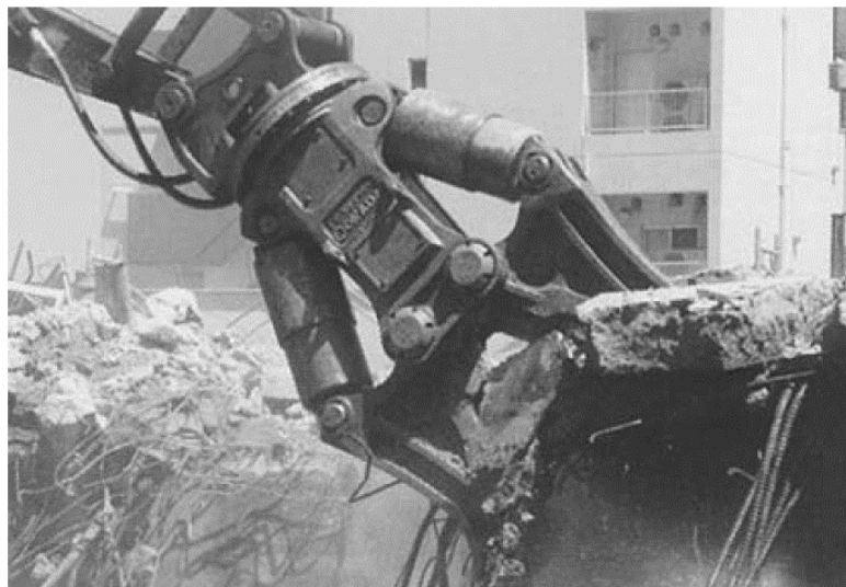
Figure 4-3 Demolition of large sections of concrete structures and buildings
