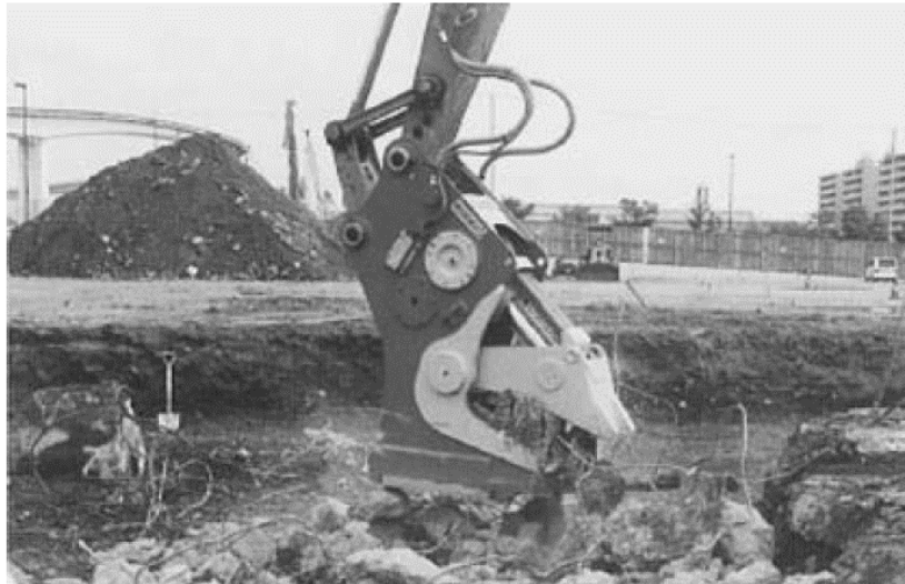
Figure 4-4 Demolition of small pieces of concrete
