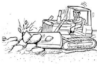
Figure 6-22 Example of pavement removal work
